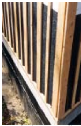
vented rain screen walls
